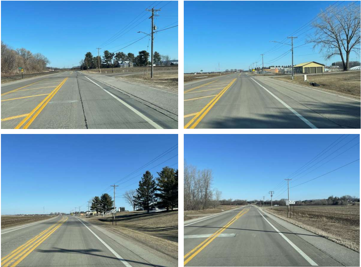
Segment B is proposed to be located along the eastern right of way of Wabasha County Road 30 from 645 th Street to Binner Way where it will connect to an existing trail.
