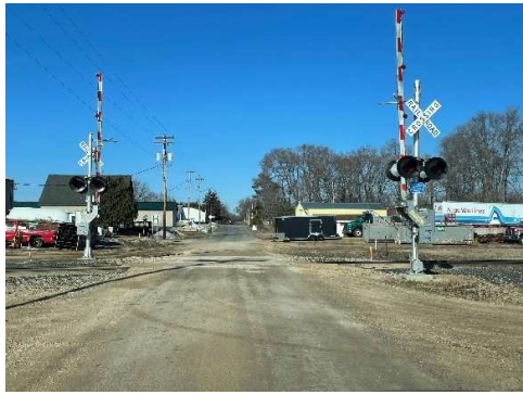
Winona Avenue Signalized/Gated Crossing of the CP Corridor (City of
